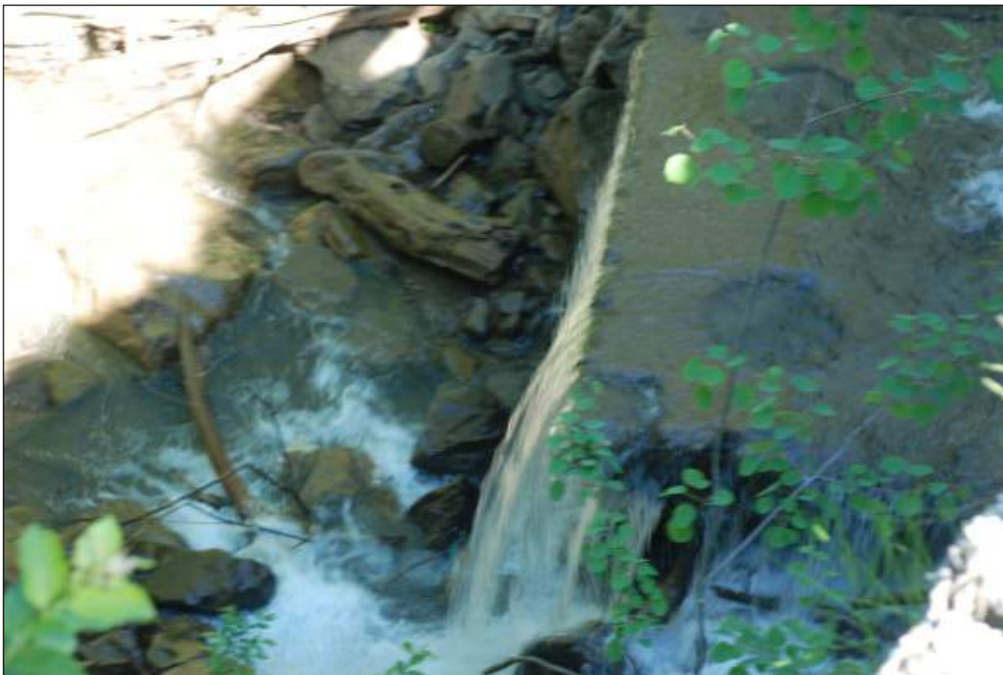
Figure 7. Concrete threshold of three m height, with no fish ladder on the upper Vişeu River.
