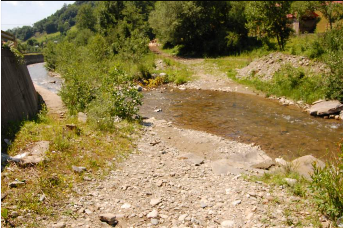
Figure 8. Frumușeaua River concrete riverbank/completely modified and road in the riverbed.
